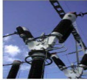
DJ12: Siemens (Type 3AQ1EE)
